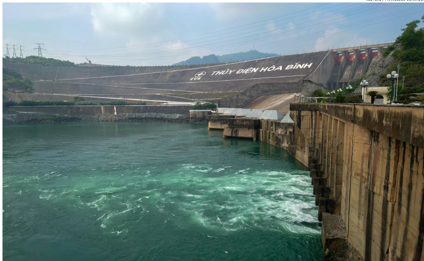
Measuring 128 metres high and 970 metres long, Vietnam's Hoa Binh hydroelectric dam is one of the largest of its kind in Southeast Asia.
